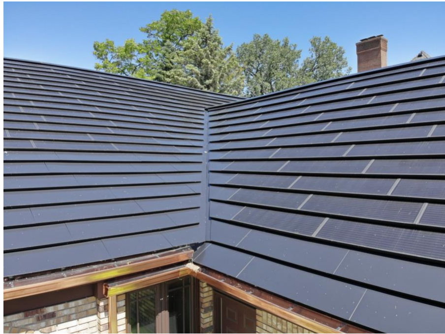
Example above of a Solar Tile installation that has a matching material at the edges that IS allowed.
