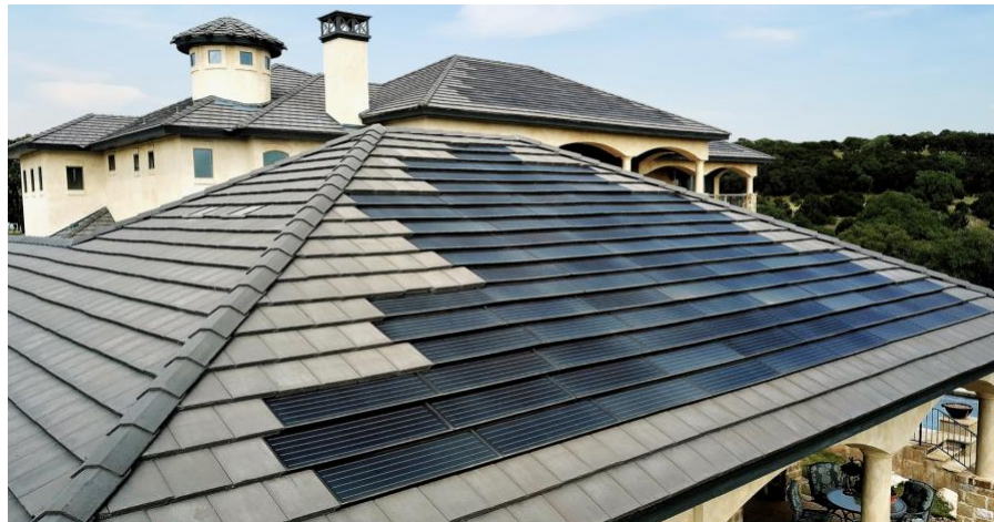
Example above of a “Patchwork” Solar Tile installation that is NOT allowed.
